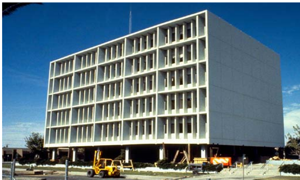
Figure 2-4 Imperial County Services Building. Earthquake damage occurred in the first-story columns at the east end of the building (photo right) (NISEE, 2013a, Collection Godden J76, Bertero, 1979).
