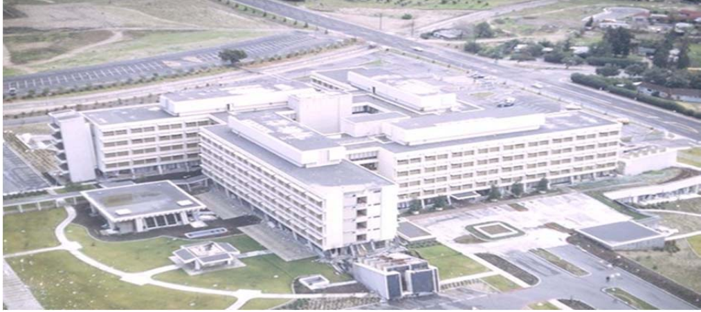
Figure 2-5 Olive View Medical Center Main Building earthquake damage (Steinbrugge Collection, NISEE, 2013b, Image S4007).
