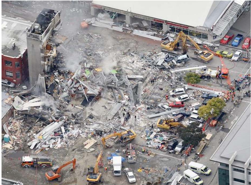
Figure 2-2 CTV Building earthquake damage (New Zealand Herald, 2011).
