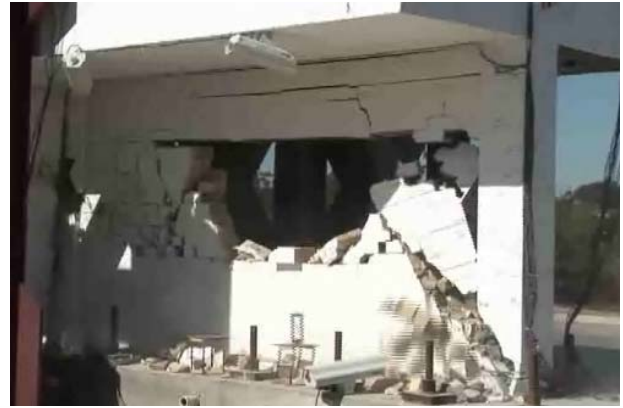
Figure F-6 Collapse of masonry infill with a window opening in a shaking-table test (Stavridis et al., 2012).
