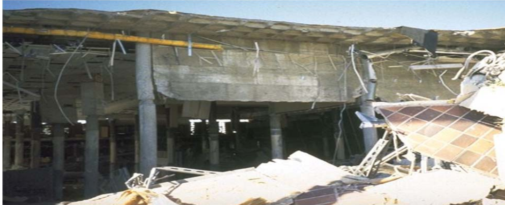
Figure 2-1 Bullock's Department Store earthquake damage (NISEE, 2013a, Photo NR222).
