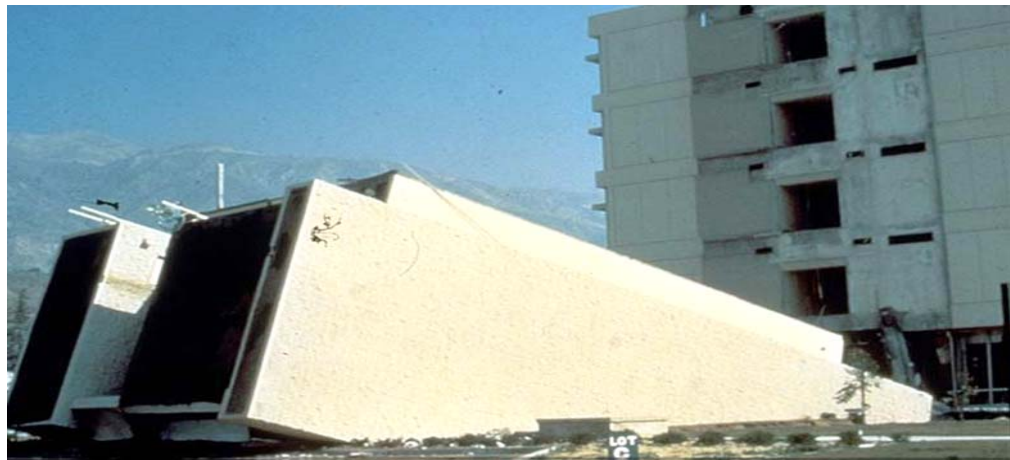
Figure 2-7 Olive View Stair Towers earthquake damage (NISEE, 2013a, Robert A. Olsen Collection, R0441).
