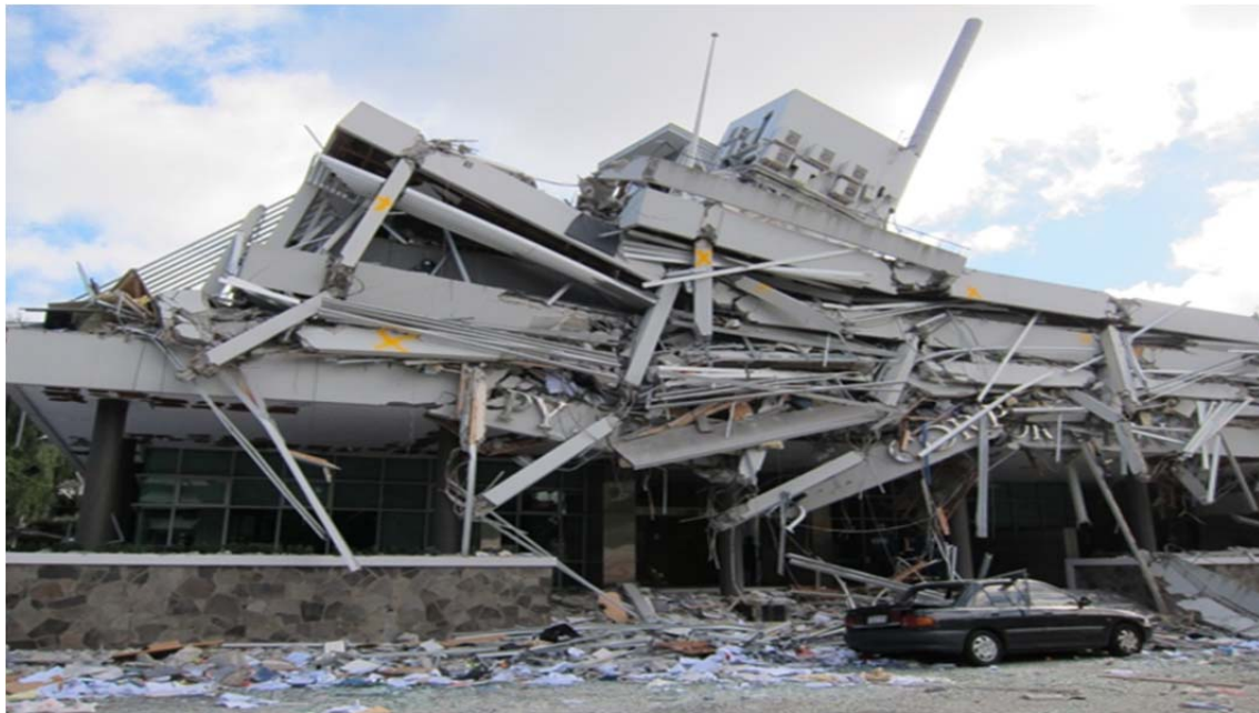
Figure 2-8 Pyne Gould Building earthquake damage (Elwood, 2011).
