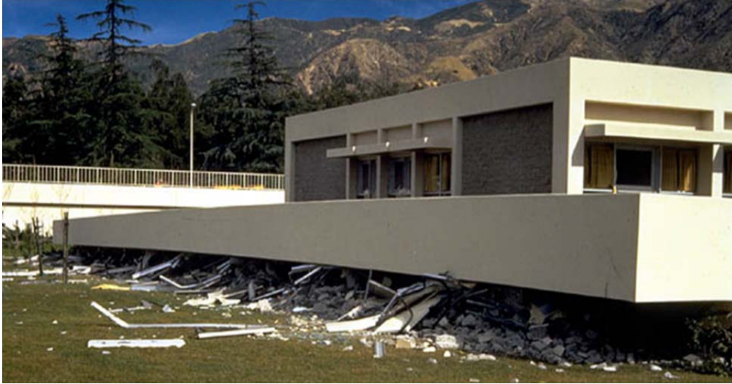
Figure 2-6 Olive View Psychiatric Clinic earthquake damage (NISEE, 2013a, Collection Godden J74, Bertero, 1971).
