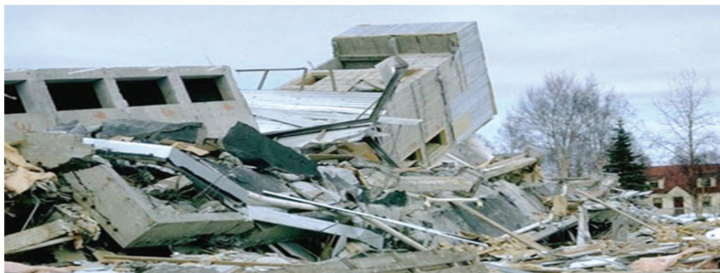
Figure 2-3 Four Seasons Apartment Building earthquake damage (Steinbrugge Collection, NISEE, 2013b, Image S2214).
