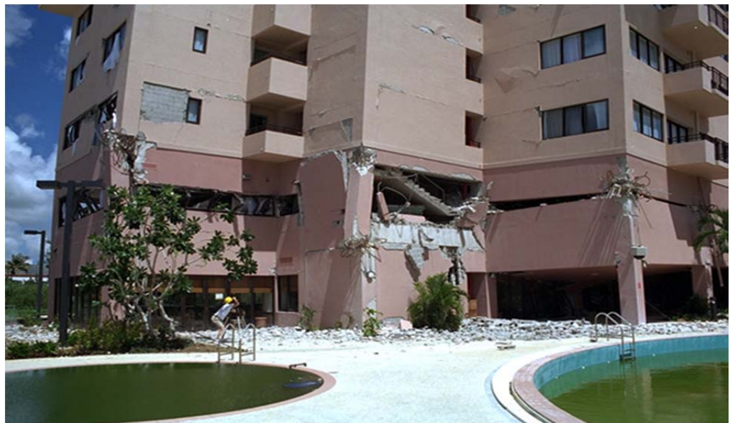
Figure 2-9 Royal Palm Resort damage (Moehle, 2003).
