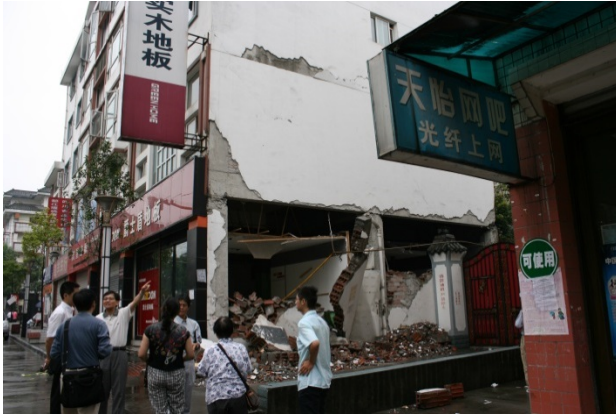
Figure F-5 Collapse of masonry infill in 2008 Wenchuan earthquake (courtesy of P. Shing, with permission).
